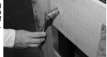
Removing skid from bottom of cabinet.
